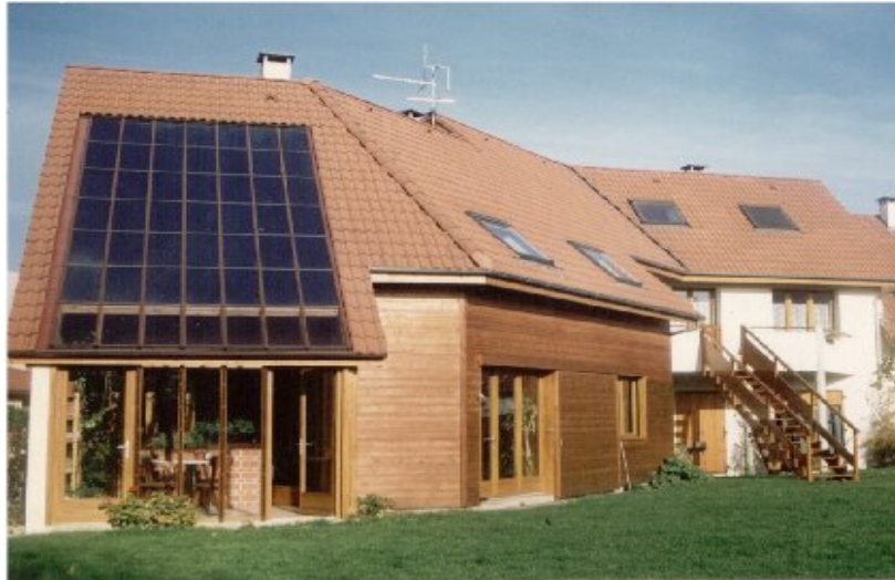
Fig. 2.12. An example of solar water heating system: solar collectors are integrated in the roof of the house directed to the south.
